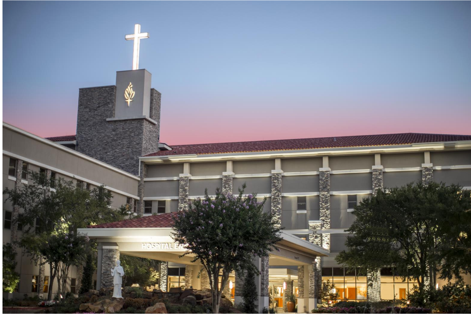
Saint Francis Hospital South 2015
